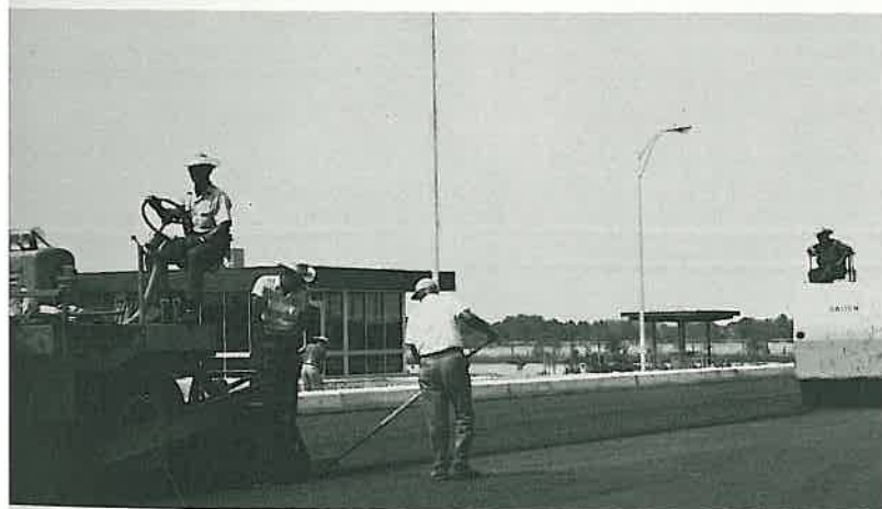
New roadside park on U.S. 67 north of Corning
