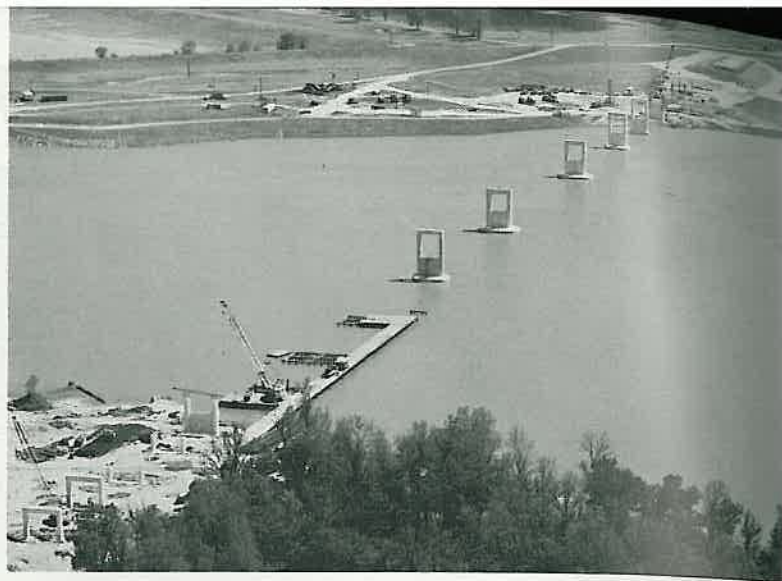
Pier construction on Pendleton bridge
