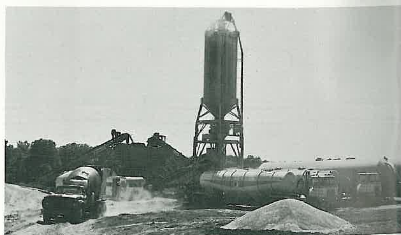
Contractor's batch plant for paving of job, top left
