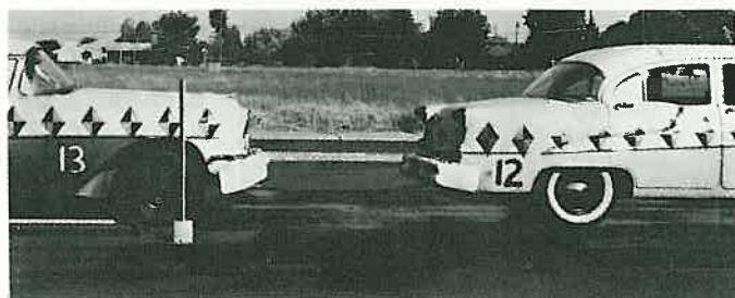
Results of a vinyl against vinyl impact at 18 mph.
