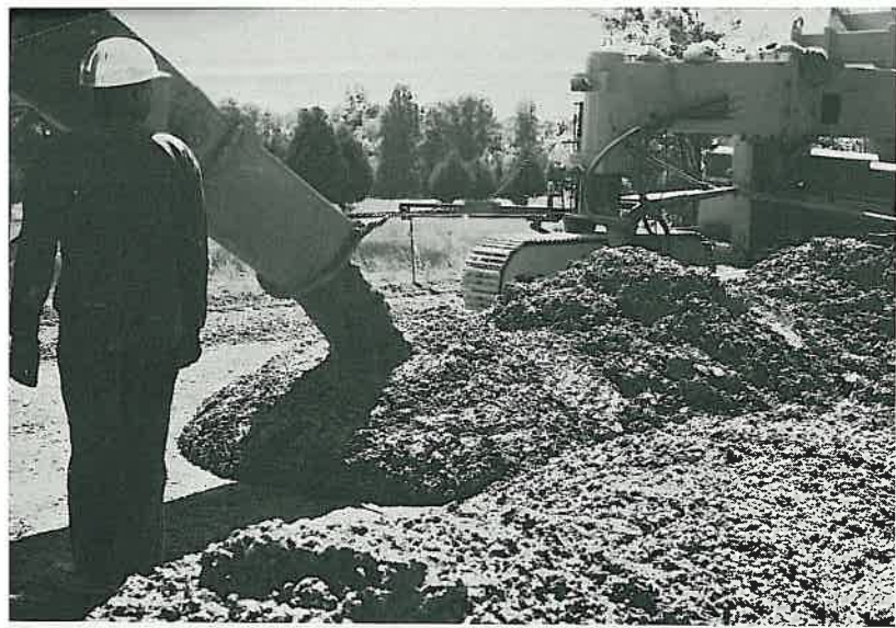
Paving on I-40 east of Russellville
